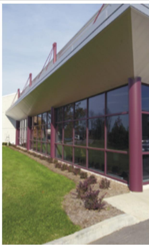
RESEARCH STATION BUILDING
